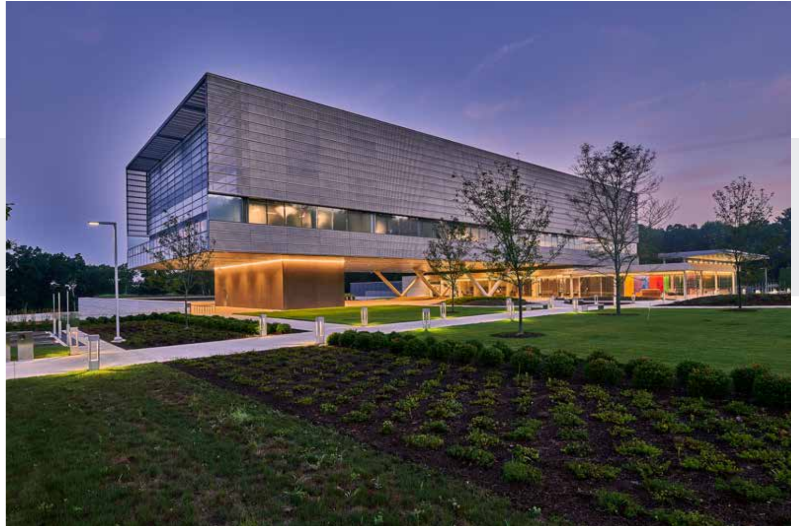
Lighting elements provide a layered approach using appropriately scaled lighting for the building for pedestrians along the path ways. Note the evenness of the lighting and minimal glare.
